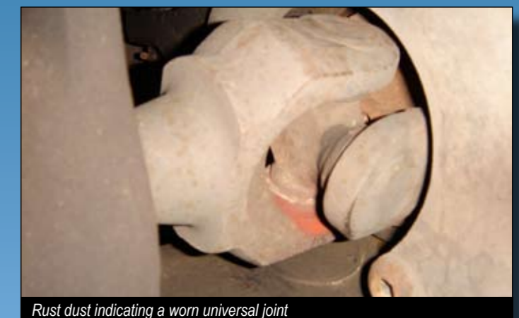
Rust dust indicating a worn universal joint
